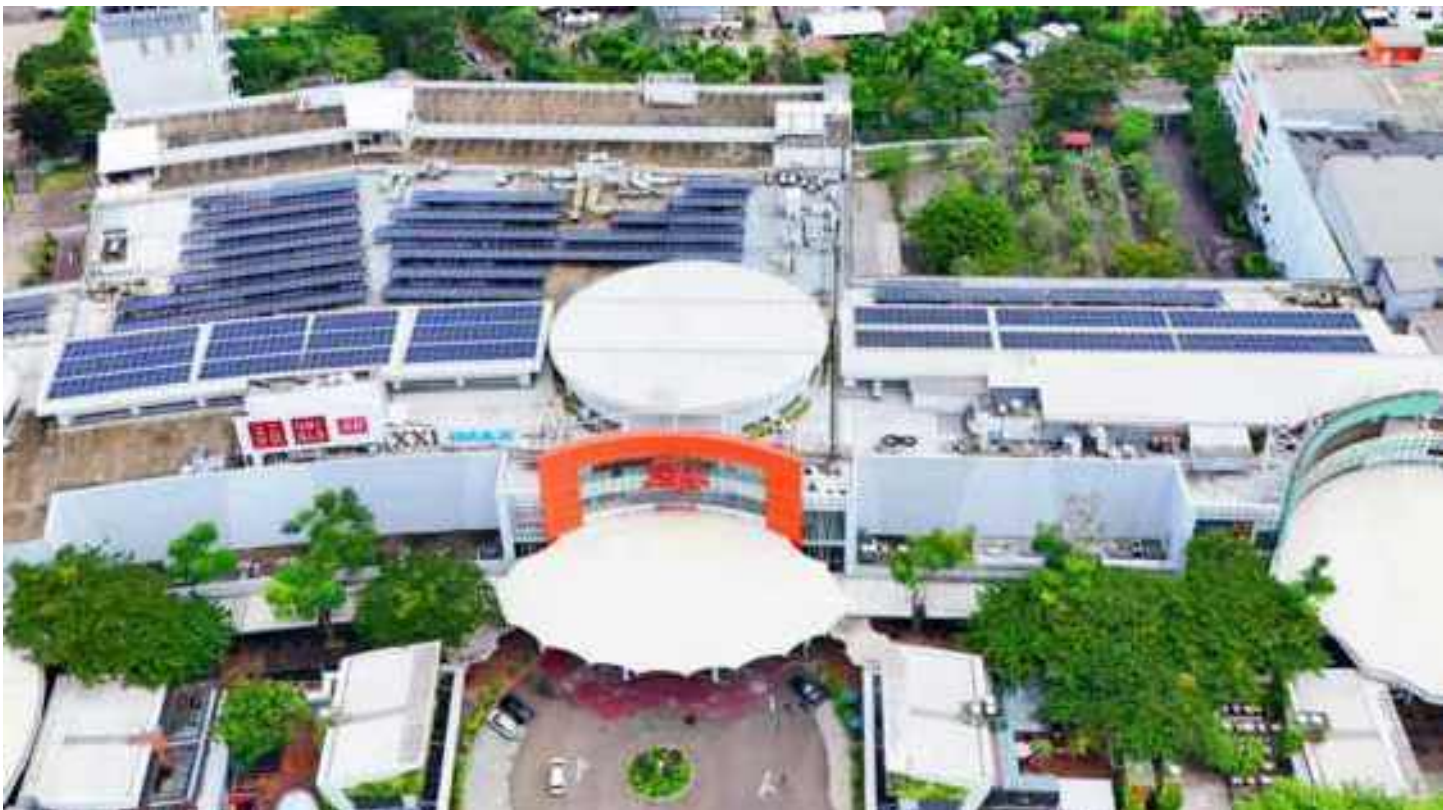
Solar panel, Summarecon Mall Serpong
